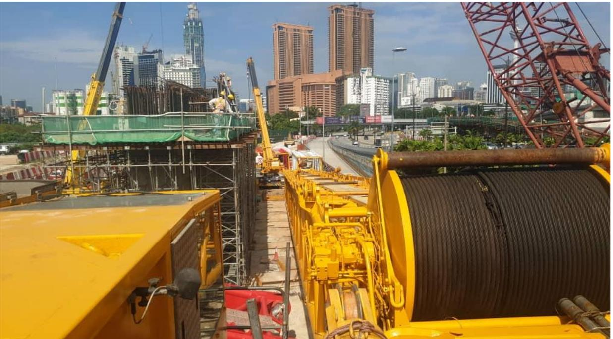
Due to the large truss dimensions, our team experienced several blind spots between the crawler crane and truss. It was one of the most challenging lifts that our Malaysia team had encountered. This was overcome by the clear communication between the crane operator and the lifting crew.
