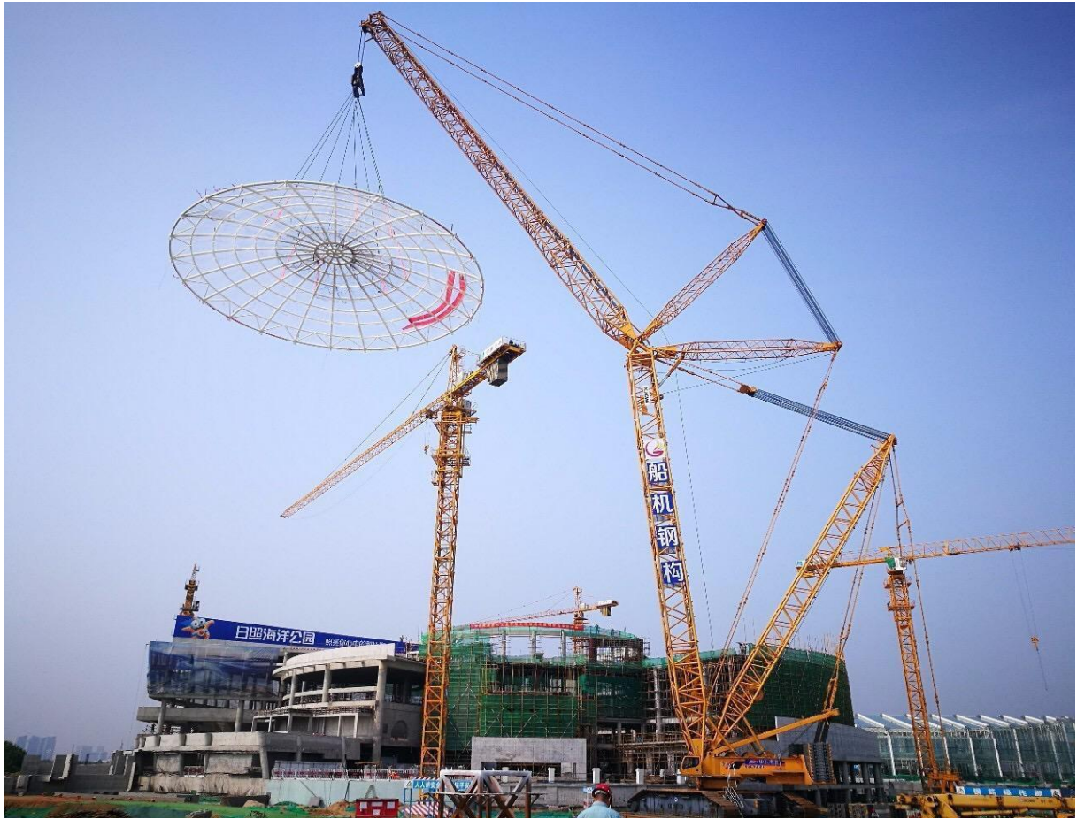
XGC16000 crawler crane helps lift the dome of rizhao oceanarium
