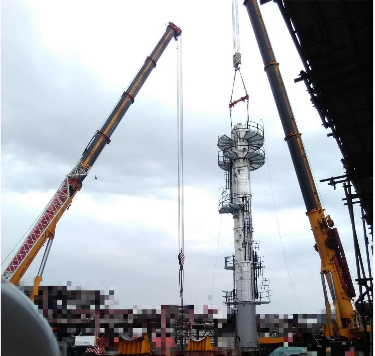
For the tandem lifting of Module 3, we deployed our Demag AC500-2 (500 Tons) and Grove GMK6300L (300 Tons).
