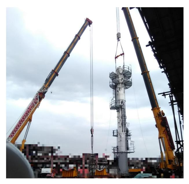
For the tandem lifting of Module 3, we deployed our Demag AC500-2 (500 Tons) and Grove GMK6300L (300 Tons).
