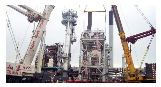
Our Demag AC500-2 (500 Tons) and AC700 (700 Tons) Mobile Cranes were deployed and configured in HASSL (Main Boom Side Superlift) for the tandem lifting of Modules for the heavy lifting operation.
